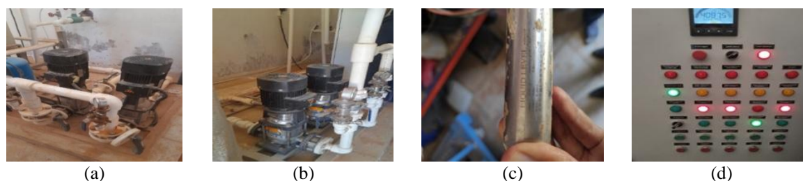
Figure 4. Moto-pumps used in water production: (a) water production pump, (b) potable water pump, (c) water level measurement is facilitated by the use of a liquid level sensor, and (d) command board
