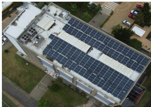
Figure 2. Roof-mounted PV plant
