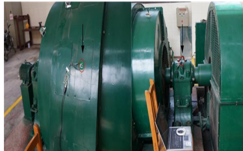
Figure 2. Wireless vibration MEMS sensors in fields
