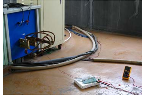
Figure 11. Mutual Inductance Electrical Transformer
