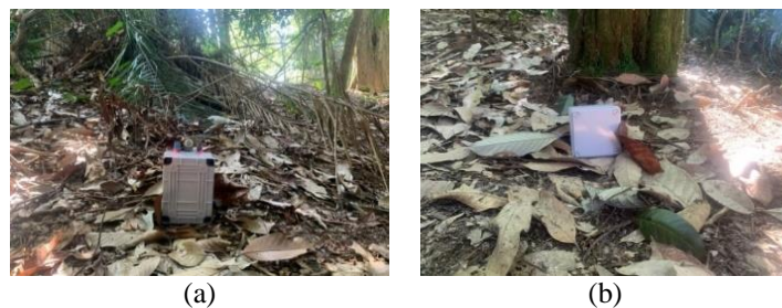
Figure 4. The placement of (a) a fire detection device and (b) a gateway in the forest community Shah Alam
