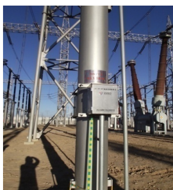
Figure 10. Monitoring Terminal on CVT Figure 11. Monitoring Terminal on PT
