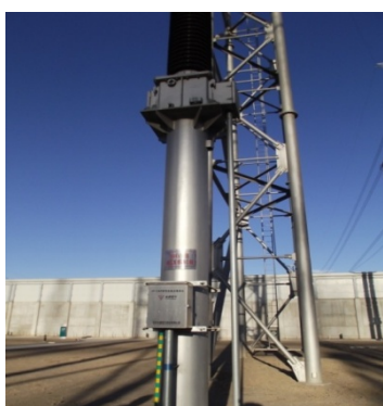
Figure 10. Monitoring Terminal on CVT Figure 11. Monitoring Terminal on PT
