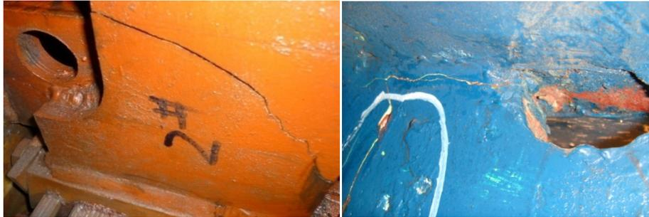
Figure 1. Generator Rotor Stand and Runner Chamber Cracks
