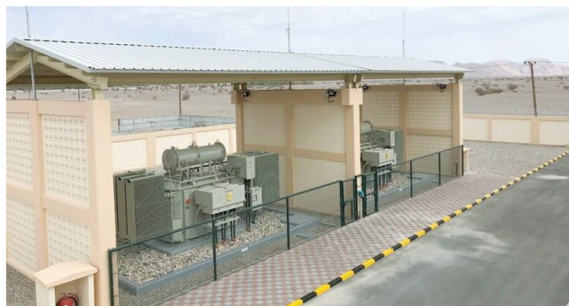
Figure 1. Al Suwairah PSS shed roof
