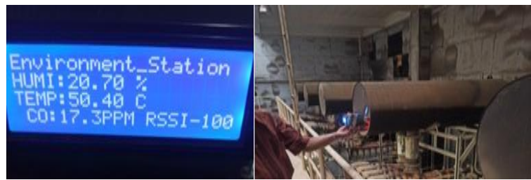
Figure 9. During the measurements in the generator room
