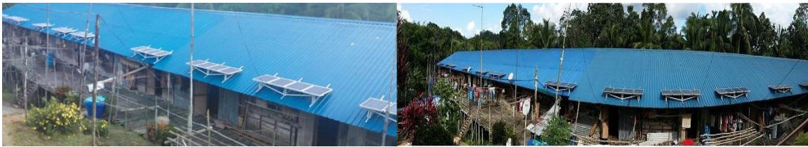
Figure 1. Installed solar PV systems at longhouse in Sarawak [8]
