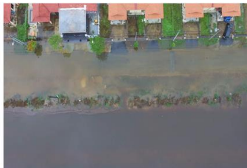
Figure 2. Flooded residential area captured by UAV
