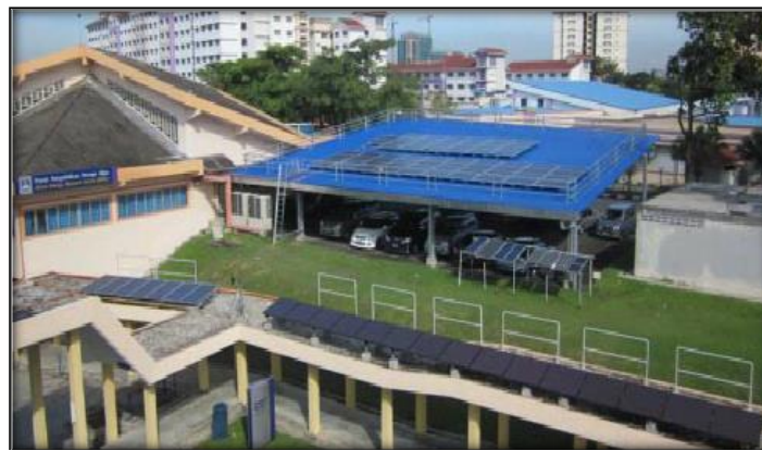
Figure 1. GCPV system test site at GERC, UiTM Shah Alam, Malaysia
