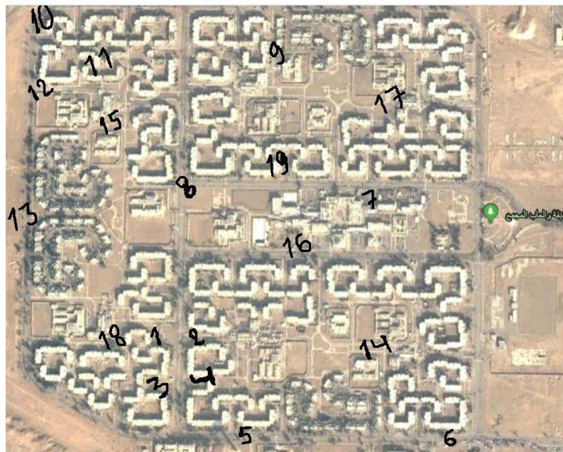
Figure 1. Top view of the Al-door residential complex
