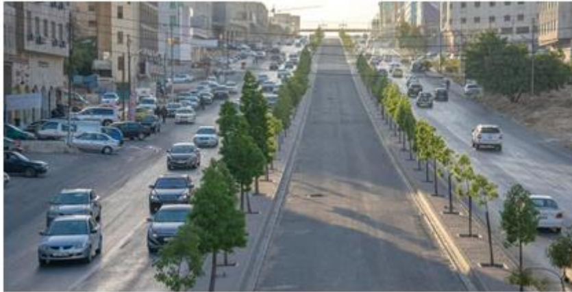
Figure 1. A view of Amman Express Bus Project
