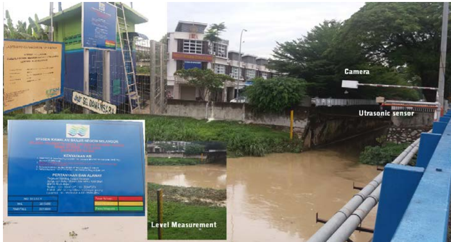
Figure 2. The Mechanism Taken by DID to Overcome Flood issue in TTDI Jaya
